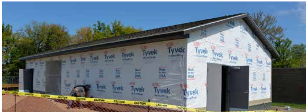
Located behind Parkside Elementary, the new storage shed for the school and district-wide maintenance is almost complete.
